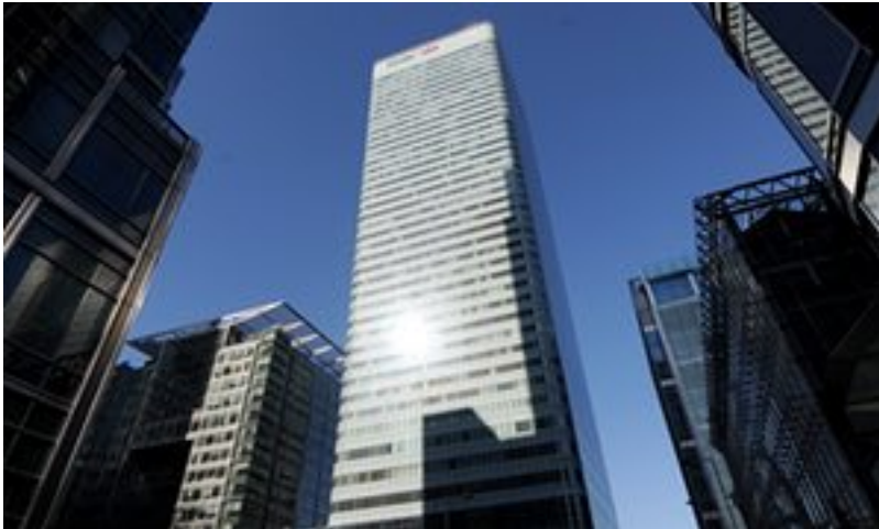
HSBC's building in Canary Wharf, London. Photograph: Anthony Devlin/PA Archive/Press Association Ima
