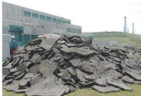
A mountain of stripped asphalt within the grounds of Kashiwazaki-Kariwa Nuclear Power Plant, after suffering damage by the Chuetsu Offshore Earthquake (July 16, 2007). Photo: Mitsuhiro TANAKA, science writer
